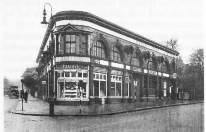
The imposing station at Chalk Farm is one of the best examples of a station designed by another well respected architect Leslie Green
